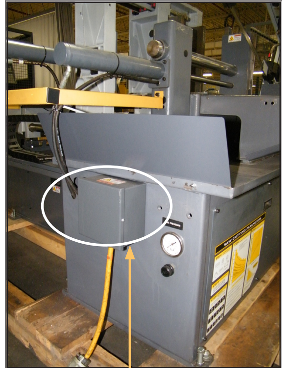
Power junction box
